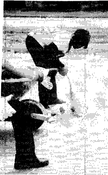
Figure 24. Using an internal vibrator
