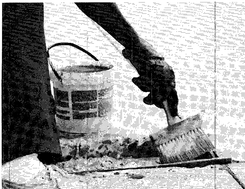
Figure 22. Applying bonding agent
