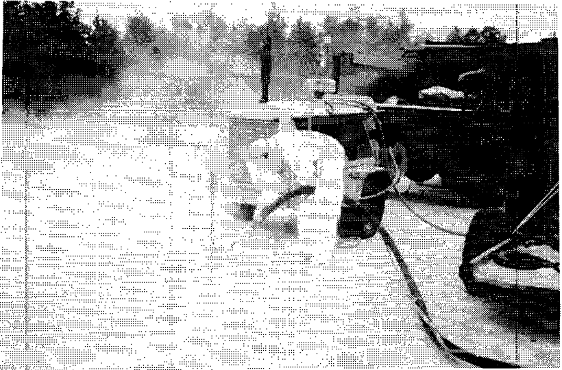
Figure 17. Sandblasting
