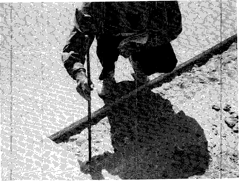
Figure 14. Sounding repair area with a steel rod
