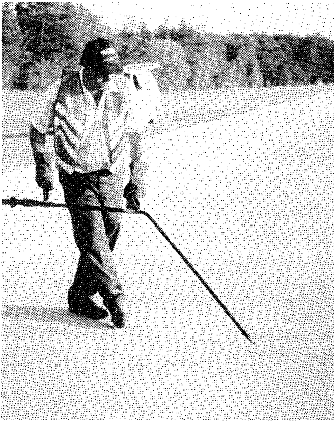
Figure 16. Hot-applied sealant installation
