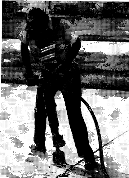
Figure 13. Using a jackhammer
