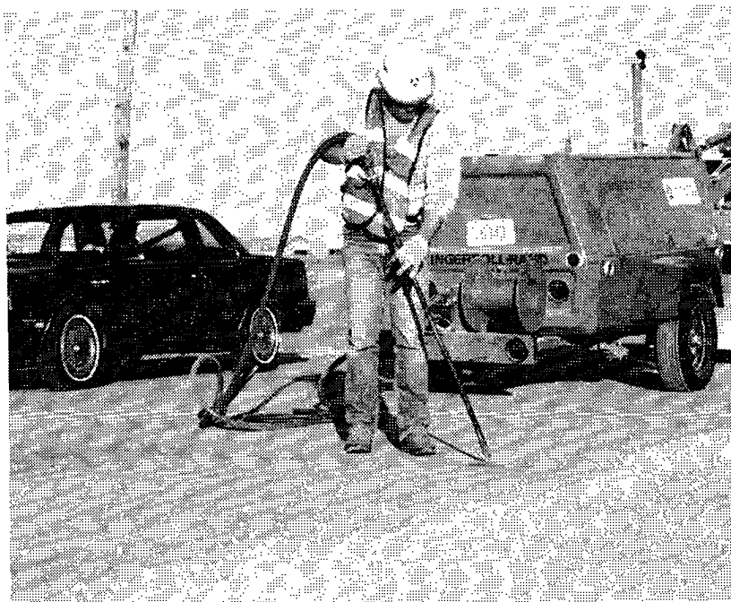
Figure 14. Airblasting operation
