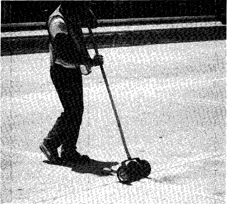
Figure 15. Backer-rod installation
